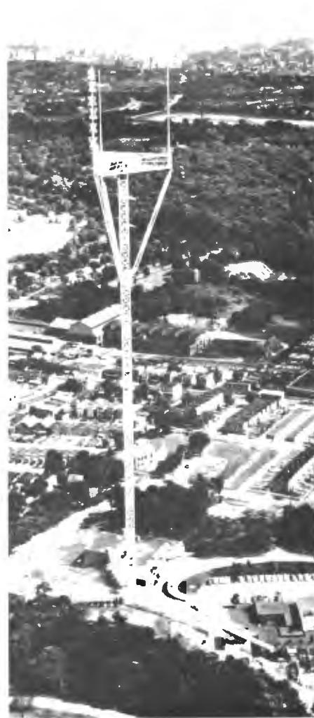
FIG. 5. The "Baltimore" candelabra was the second such tower. 725 feet tall, the tower "sees" virtually every part of the Baltimore metropolitan area. Supporting two RCA Traveling-Wave Antennas and an RCA Superturnstile, the tower is now being extended to 1000 feet.
