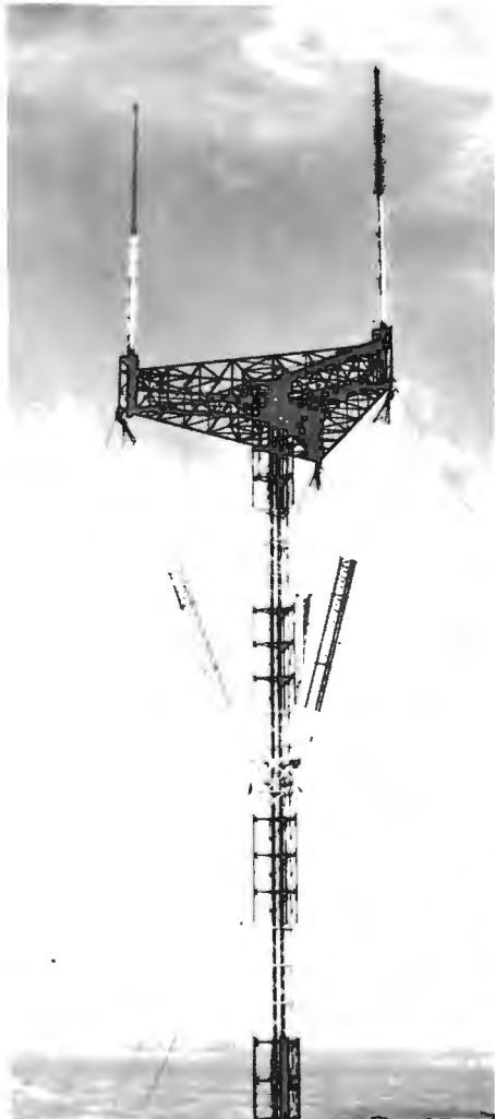
FIG. 4. The "candelabra" antenna tower extends tower usefulness by placing all antennas at the same level. This tower, the "Dallas Candelabra," was the first of the "birthday-cake" towers. The tower now supports two TV antennas as shown here plus two "interlaced" FM antennas.
