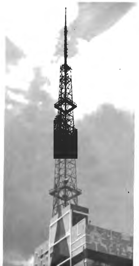
FIG. 22. As this article was being written, Mexico City installed a diplexed superturnstile for Chs. 4 & 5. It's a four-section S-T on top of a four section Ch. 2 superturnstile. This photo shows the self-supporting tower as a background for one of the buildings of Telesistema Mexicana, Mexico City.
