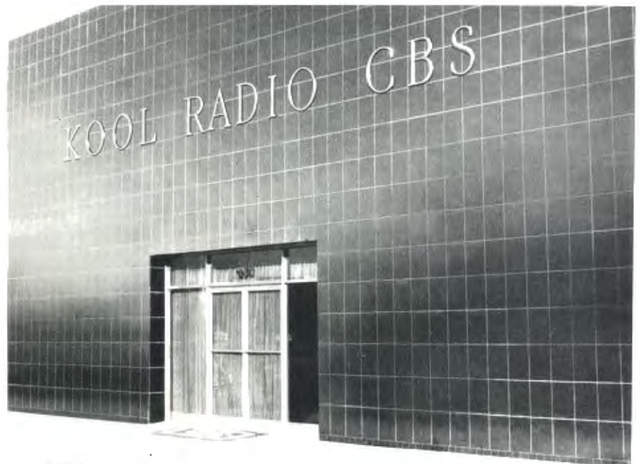
FIG. 1. KOOL's street-front building is finished in bronze ceramic-veneer tile with red lettering. The metal framing of the portico is gold-anodized to harmonize with the bronze-colored tile.
