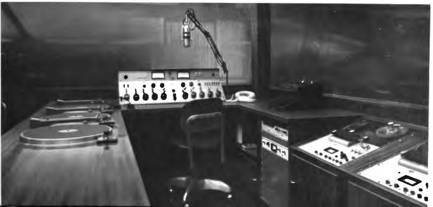
FIG. 5. Production Control is arranged very much like Master Control except that there are two reel-to-reel tape machines (RT-21) and one tape-cartridge system equipped with recording facilities.
